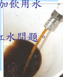
The manganese in the treated water oxidized in the distribution system and resulted in black-brown water at the tap.
